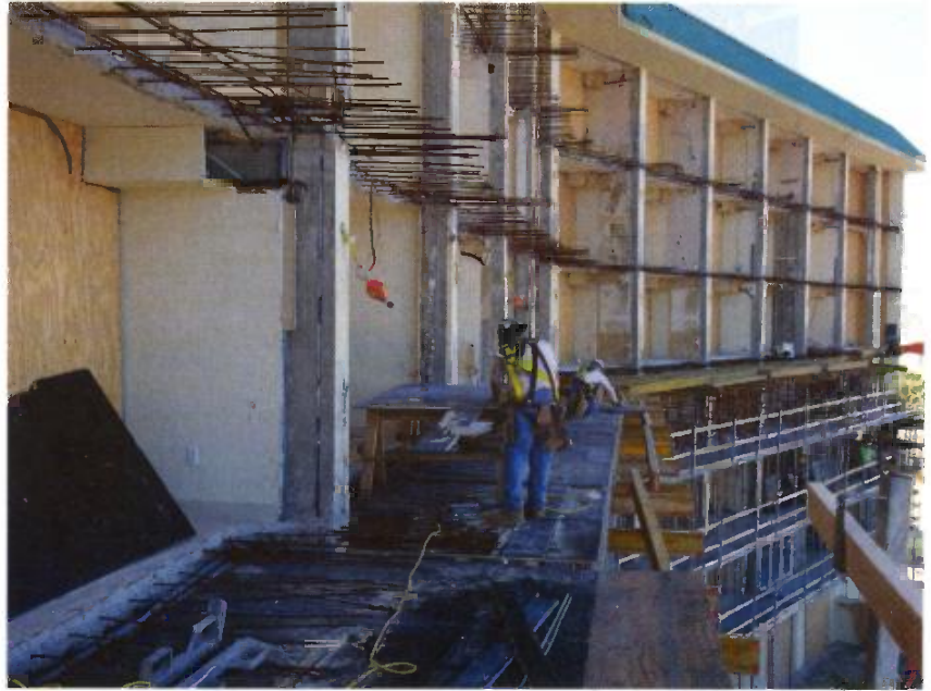
Work proceeding on balconies
