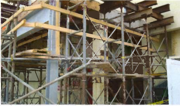
Replacement structural steel columns and beams
