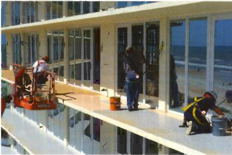
Coating being applied to new balconies
