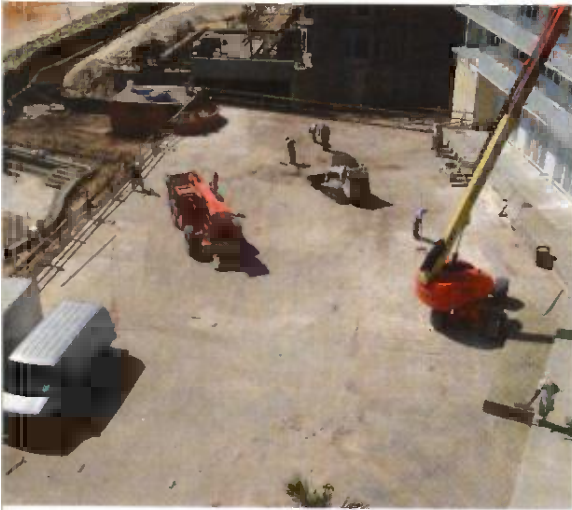
Work proceeding on new deck and pool area
